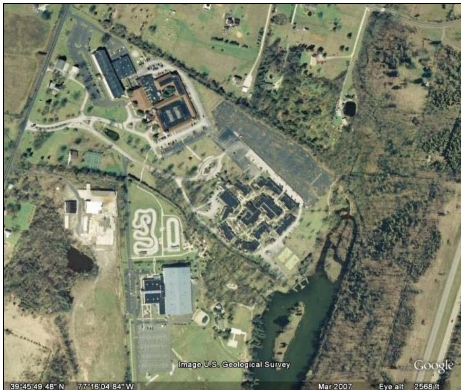
Figure 1.5.1 Aerial Photograph of Existing Eisenhower Hotel & Conference Center
