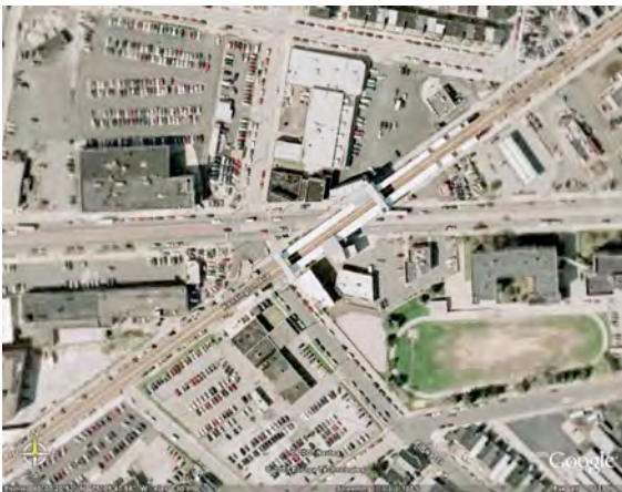
Figure A.3 – Erie-Torresdale Avenue MFL Station
