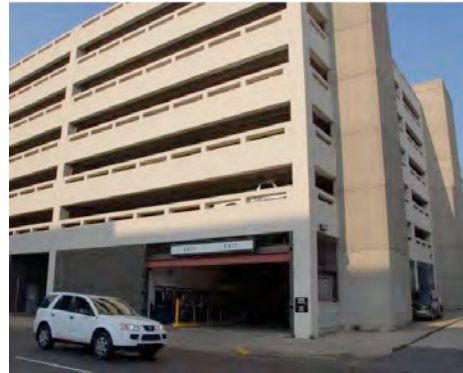
9 th and Race St. parking garage with no ground floor retail
